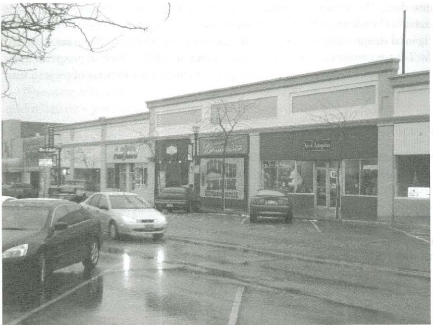
FIGURES 11.1–11.5 Examples of a community-driven design project from a Main Street program (Historic Downtown Kennewick Partnership, Kennewick, Washington) catalyzed by a facade grant program
